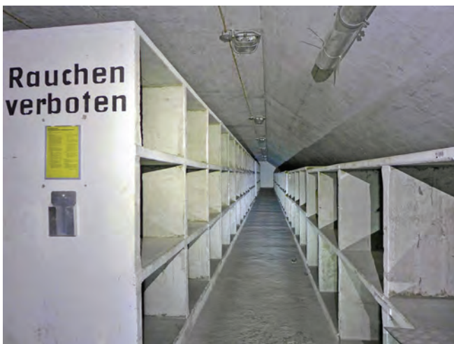
Fort Furggels: One of the magazines for the 10.5cm turret guns. The roof profile is characteristic of the concrete structures of this period built within excavated chambers. The later 15cm magazines had a larger, arched cross-section, similar to those at Fort Sasso da Pigna
